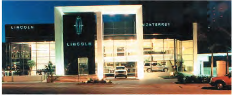
Fig. 138 Vista fachada principal
